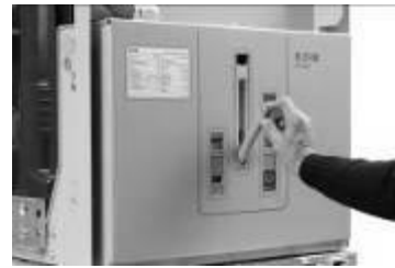
Fig. 5-1: Pull the round handle down
