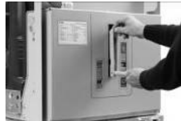
Fig. 5-2: Pull out the handle with two hands
