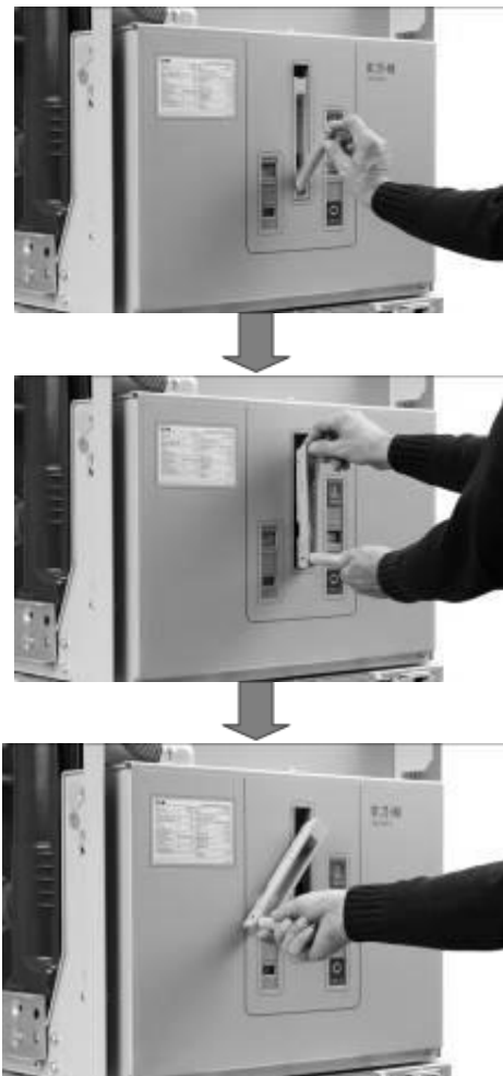
Fig. 6-5: Manual Charging Process
