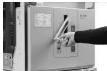
Fig. 5-3: Turn the handle clockwise
